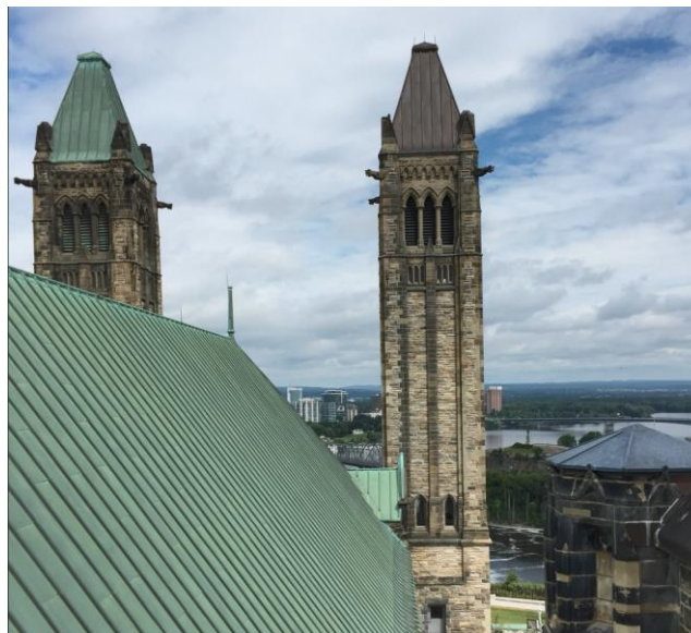
Figure 2: East ventilation tower
