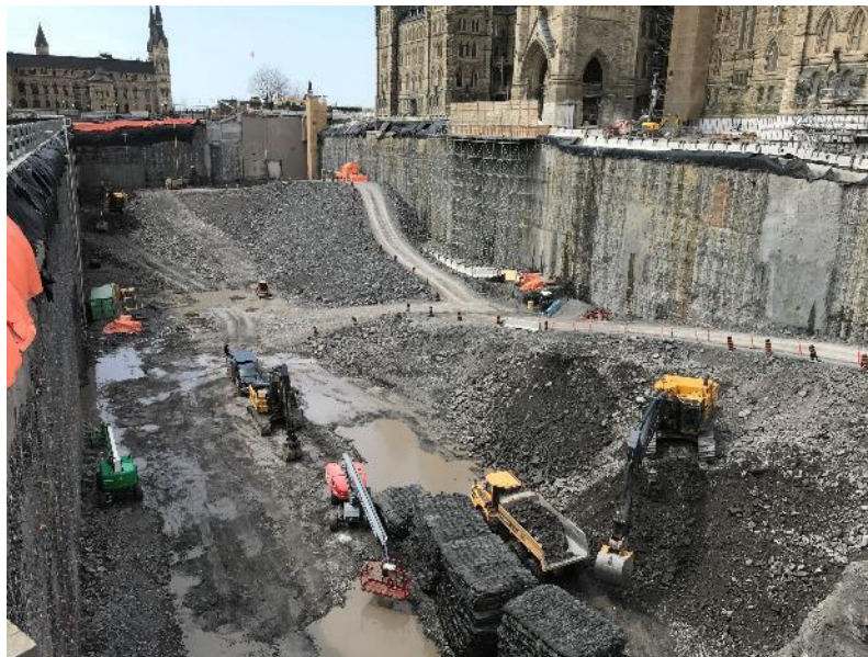
Figure 3: Centre Block's Parliament Welcome Centre excavation, April 2023
