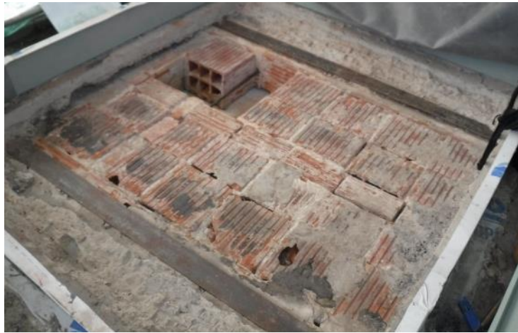
Figure 4: Hollow terracotta tile floor assembly
