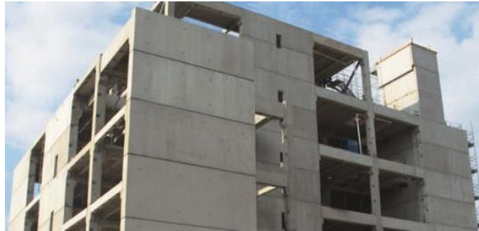
Figure 2. Precast wall panels as shear walls [2].
