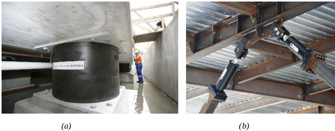
Figure 4: Examples of alternative strategies for seismic resiliency (a) seismic isolation (From Seo [6]) and (b) supplemental damping (From Taylor Devices [7])
