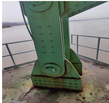
Figure 9. Pendulum anchorage at Pier 4 & 7
