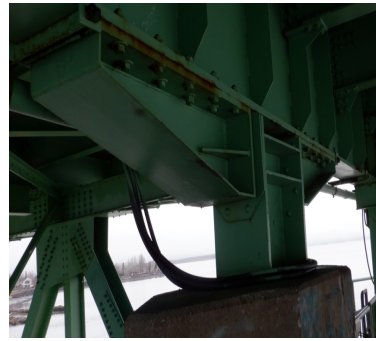
Figure 10. Wind shoe at Pier 4 & 7
