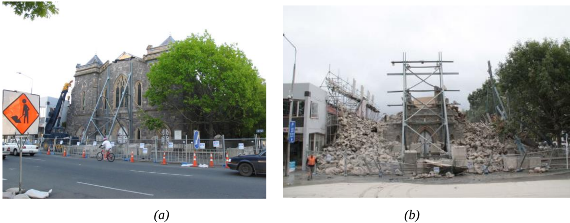
Figure 6. Photos of the Durham Street Methodist Church: (a) under reconstruction in November 2010 (Source: Robertson, 2010 [55]), (b) collapsed in the February 2011 earthquake (Source: Aldersgate Centre, 2011 [56]).
