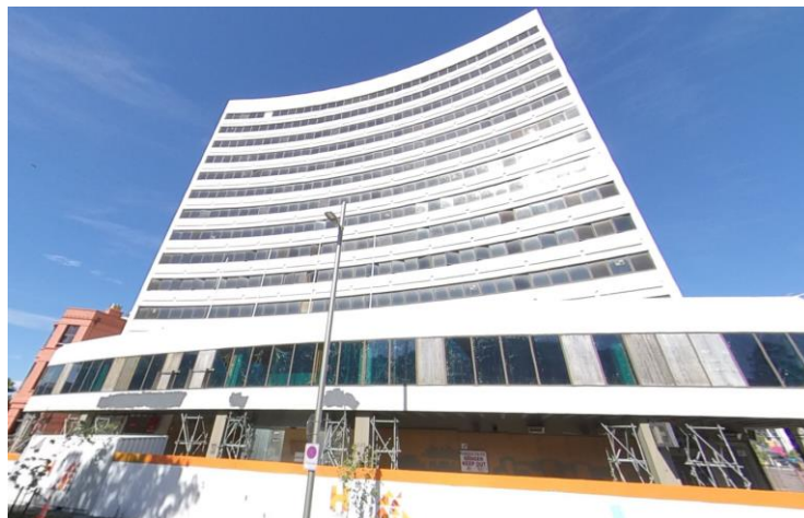
Figure 7. Photo of the 85 Worcester Street building as unattended due to insurance decisions (Source: Google Maps Street View, 2023 [57]).
