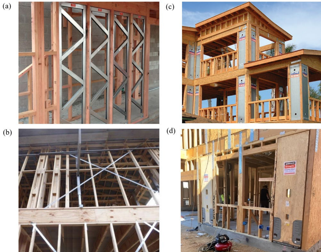
Figure 2. Samples of seismic solutions for Residential applications: a) Truss bracing by Gamma brace Ltd. [1], b) Tension-only straps, c) Steel shearwalls by Mitek Ltd. [2], and d) Timber shearwalls by Simpson Strong-Tie Ltd. [3]
