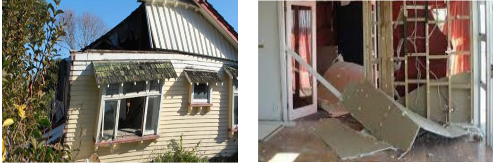
Figure 1. Samples of seismic damage to residential buildings constructed by light timber framing
