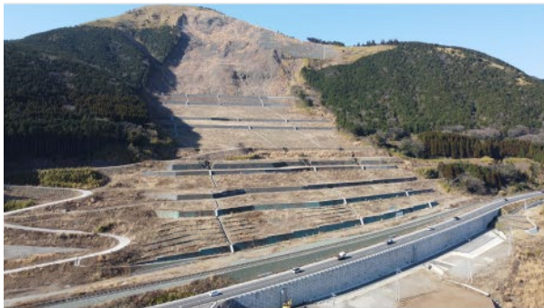
(a) Slope stability works for the largest landslide
