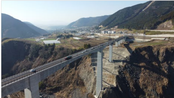
(c) Completed New Aso-Ohashi bridge
