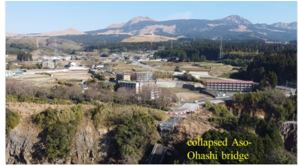
(b) Kawayo district and collapsed Aso-Ohashi bridge
