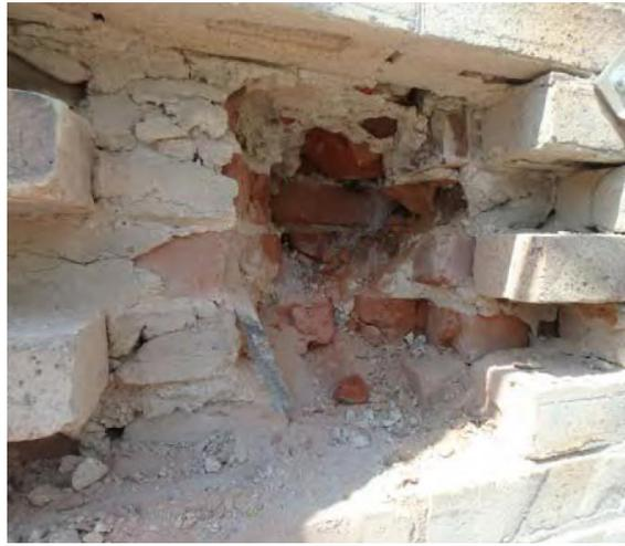
Figure 2. Building A unreinforced masonry brick load-bearing walls composition
