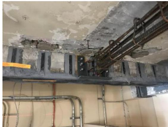
Figure 11. Collector Beam in B wing
