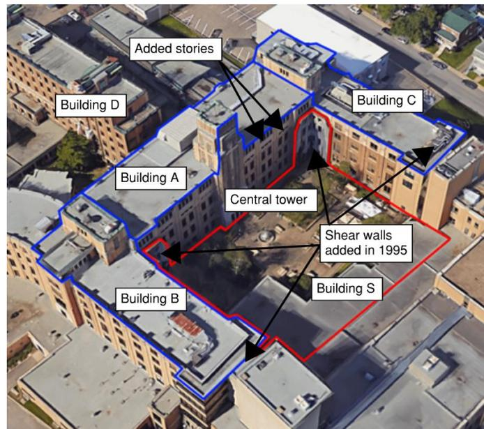
Figure 1. Construction stages of the SABC building ensemble
