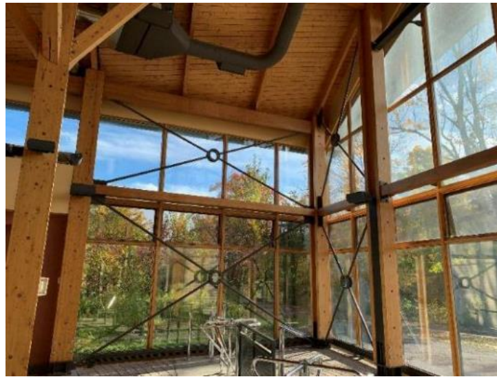
Figure 2. Existing steel bracing system.
