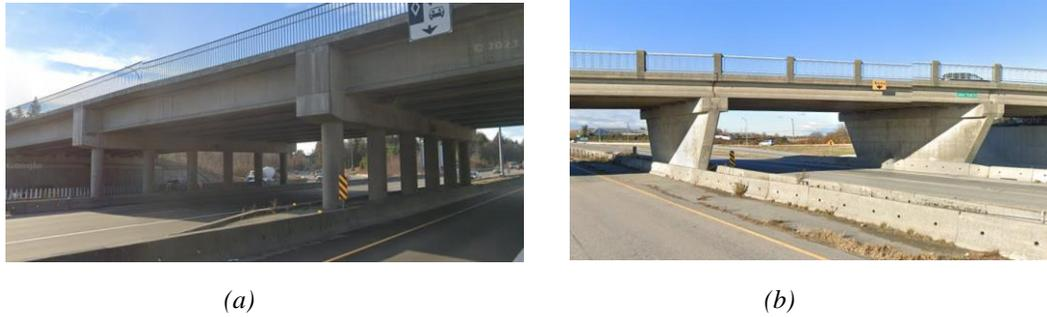
Figure 1. Sample bridges in Metro Vancouver with: (a) RC circular columns, (b) RC rectangular walls [8].
