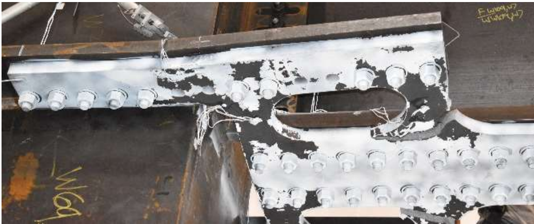
Figure 7. Ductile tearing of fuse plate of Specimen K2.2.
