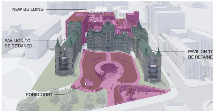
Figure 1. Overview of the New Vic Project, with the retained buildings, the new building and forecourt to be added.
