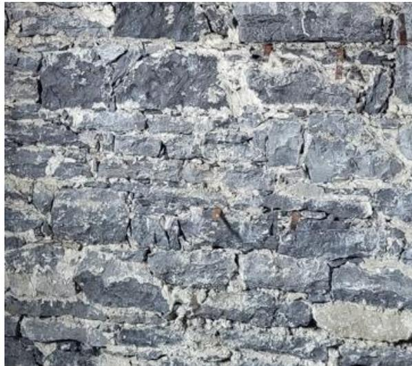
*Figure 4. View of the interior face of a rubble wall observed on site.*
