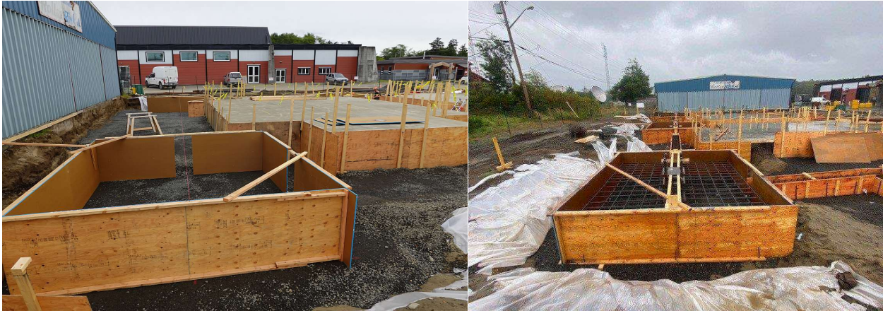
Figure 7. Foundation construction large spread footings, the construction required temporary closure of the basketball court. The photo at right is courtesy of Unitec Construction Ltd.
