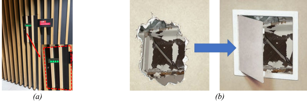
Figure 3. Access panels used for structural maintenance: (a) Access panel for MEP, (b) Proposed structural access panel (SAP)
