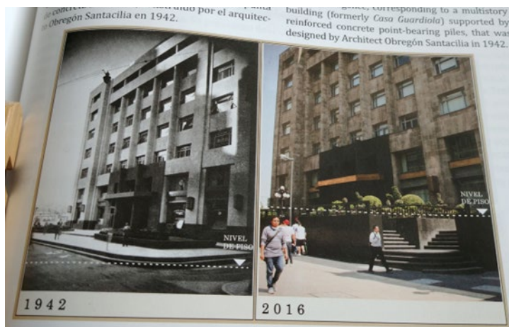
Figure 2 A building grew downward between 1942 and 2016 to adapt to the situation of ongoing settlement of surrounding ground and the building itself that is founded on piles
