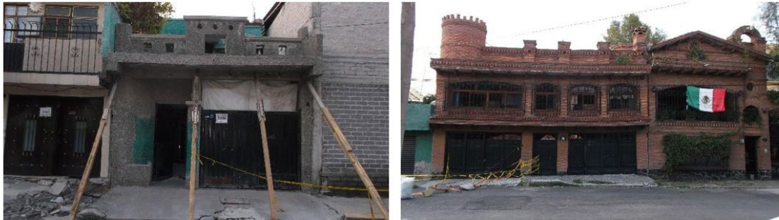
Figure 3 Buildings damaged by intensified ground settlement and crack during September 19, 2017 Puebla-Morelos Earthquake
