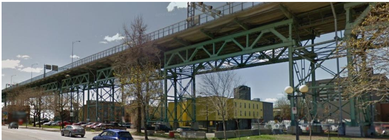
Figure 14. General view of Section 8 of the Bridge
