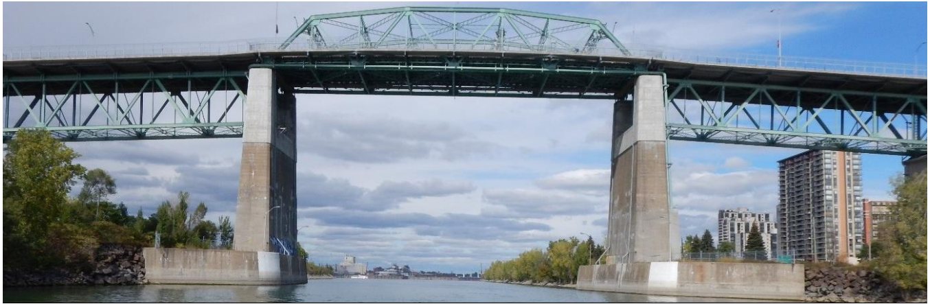
Figure 7. General view of Section 3 of the Bridge
