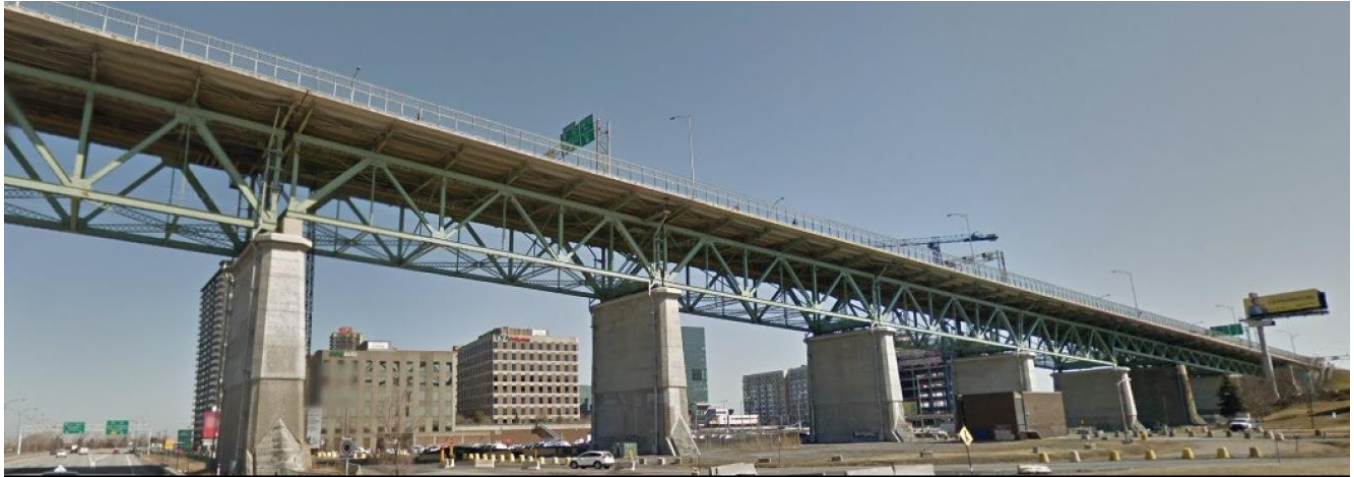
Figure 5. General view of section 2 of the Bridge (South approach)
