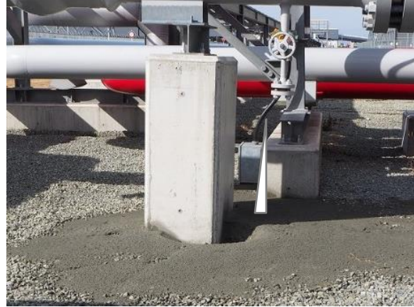
(a) Sand boiling adjacent to foundation (b) Uneven settlement of foundation with adjacent sand boiling
