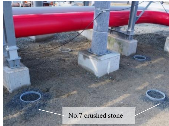
(b) Crushed stone ejected from \phi 300mm drainage pipe
