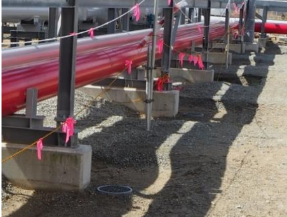
(a) Group of pipework foundations
