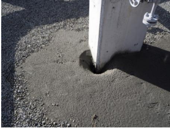
(a) Sand boiling adjacent to foundation (b) Uneven settlement of foundation with adjacent sand boiling
