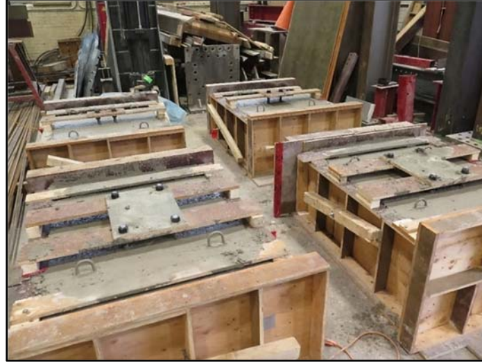
Figure 6: RC Foundation blocks post concrete casting
