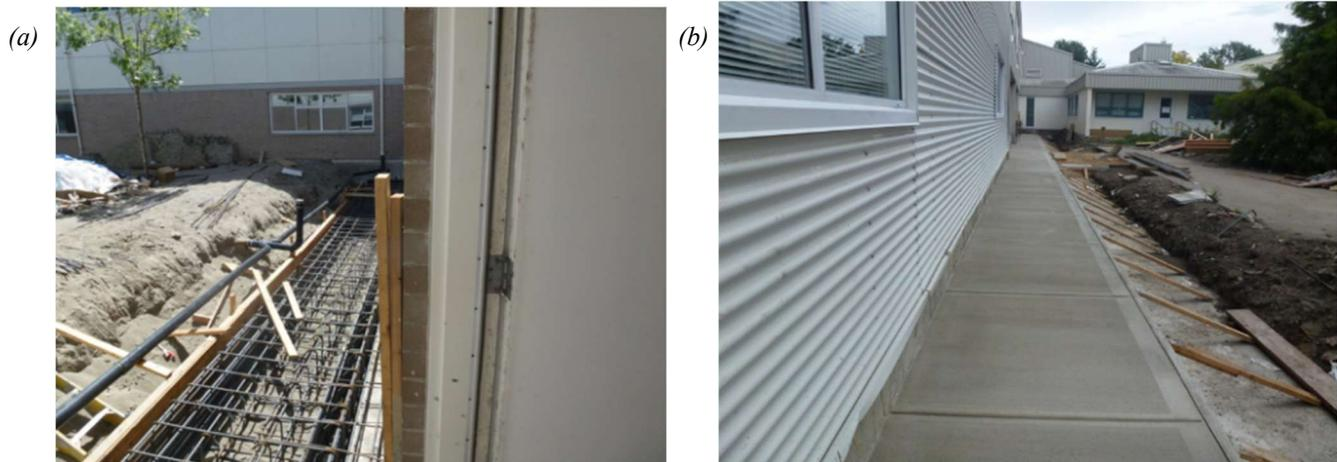
Figure 11. External Ring Beam (a) During Construction, (b) as Sidewalk When Completed
