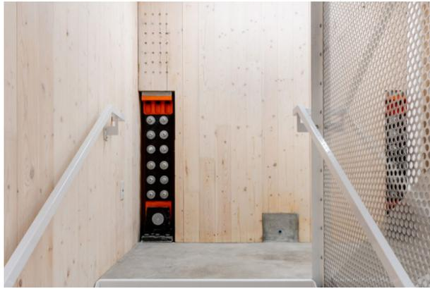
Figure 1. Photo of the installed Tectonus HD
