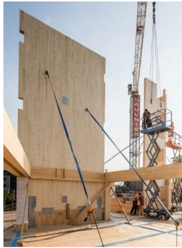
Figure 5. Balloon-type CLT building under construction (Courtesy of Nordic Structures).
