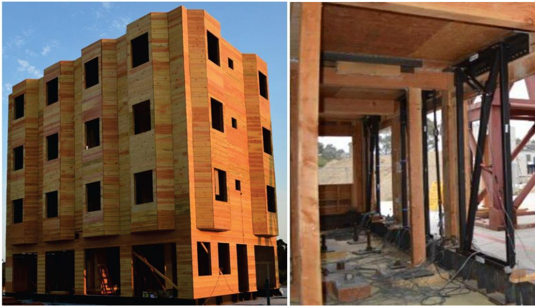
Figure 5. NEES-Soft model and toggle-braced dampers at first story [12]
