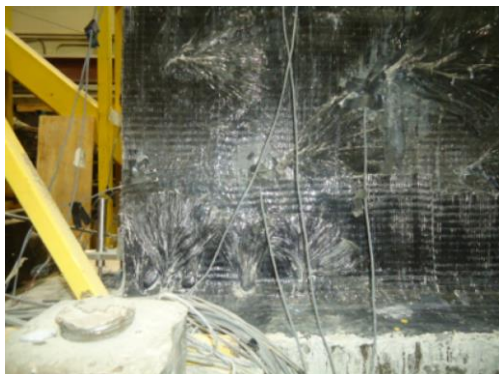
d) Close up View of Installed CFRP Anchors
