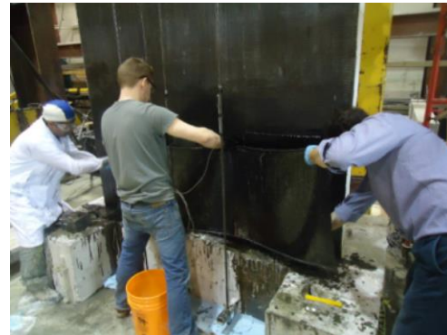
e) Anchors covered by a Layer of CFRP
