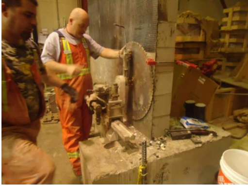
a) Cutting of the foundation concrete
