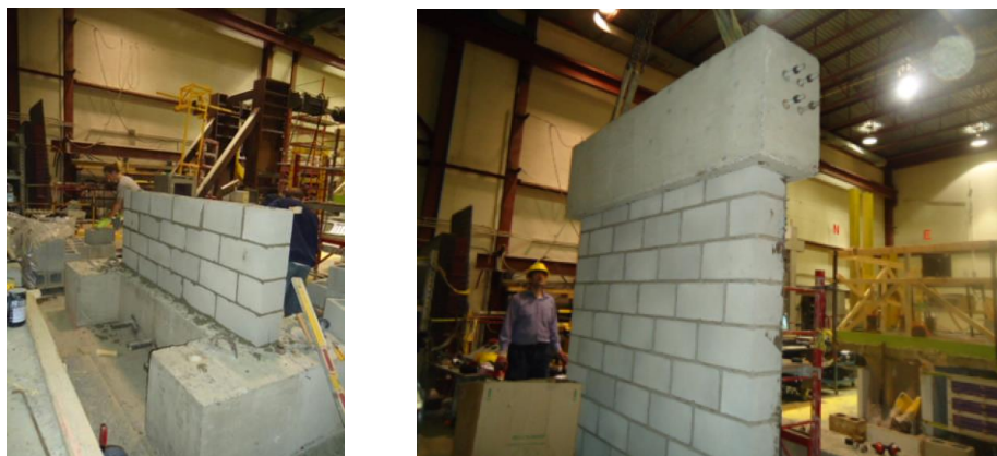
Fig. 3 – Masonry walls during construction
