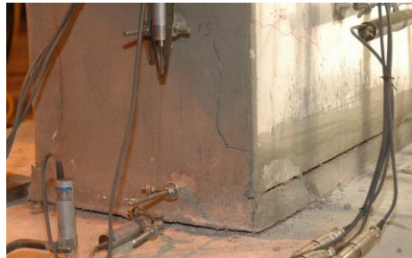
d) Observed base cracks at drift ratio of 0.5%
