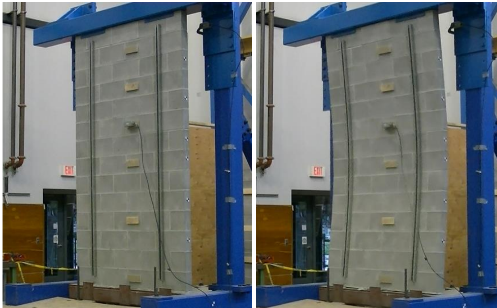
Fig. 3 – Deformed Shape of U-Channel Retrofitted Wall
