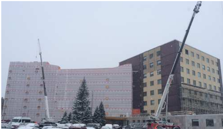
Figure 11 – East side of wing B under retrofit work
