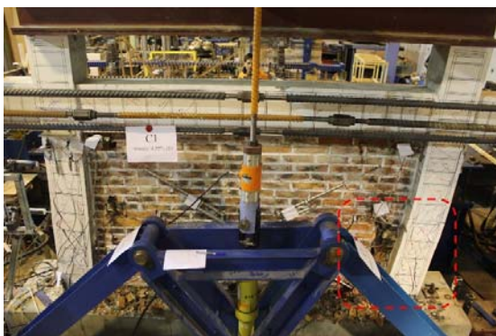
(a) short column failure of right column
