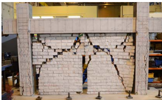
(a) overall view
