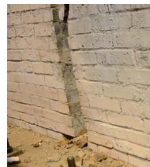
(b) integrity of infill panel
