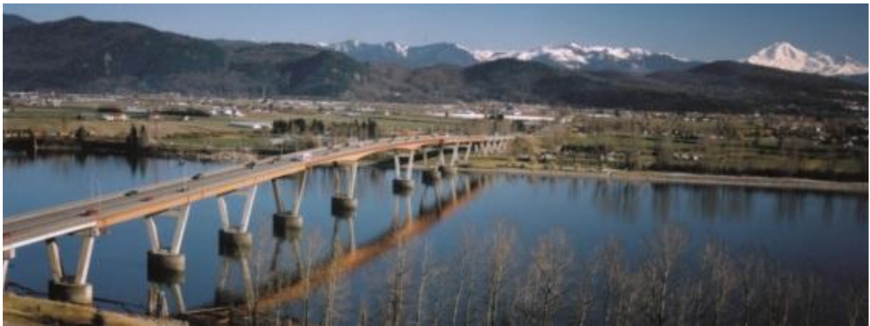
Figure 1 – Mission Bridge Aerial View Looking SE
