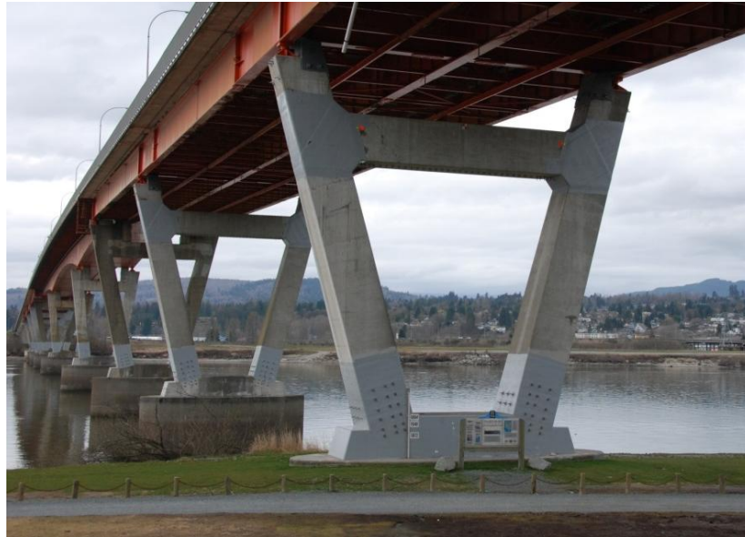
Figure 2 – Pier S4 (looking north-east ) prior to retrofit with UHPFRC jackets
