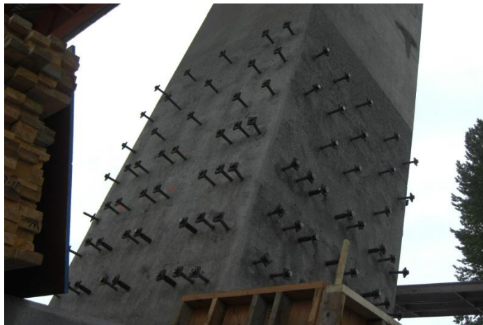
Figure 6 – Pier S4: Column preparation with sandblasting and installation of dowels
