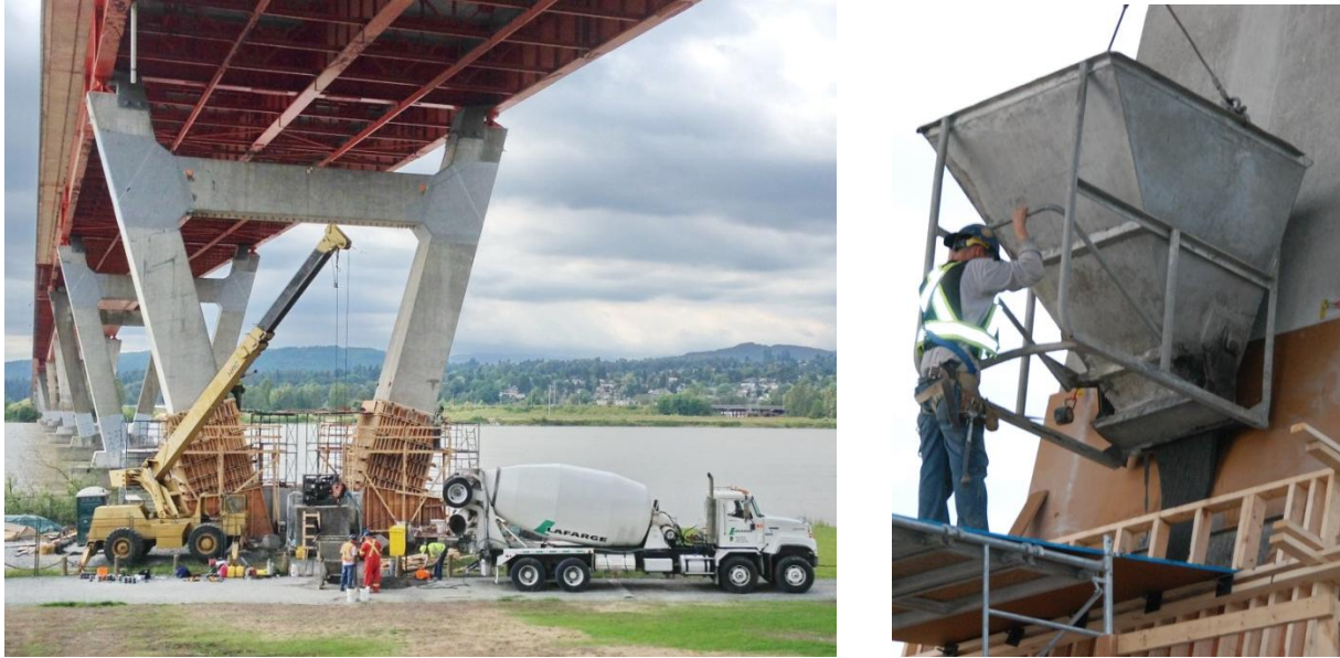
Figure 7 – Casting of UHPFRC jacket
