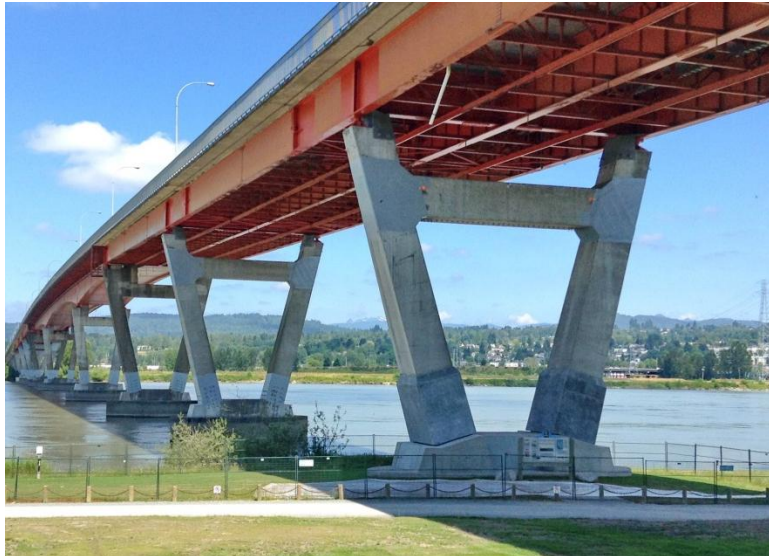
Figure 9 – Pier S4 after Completion of Construction
