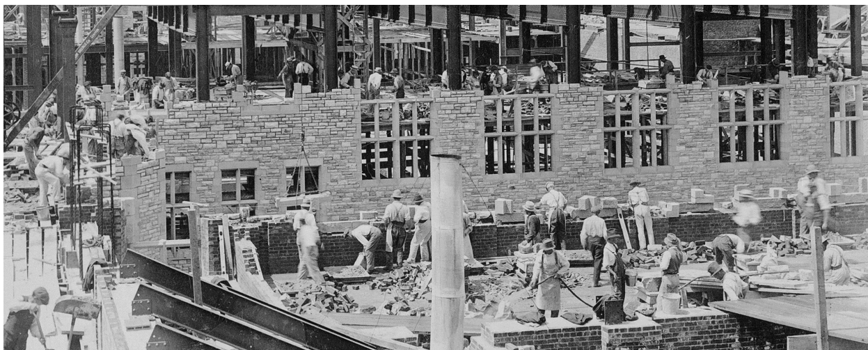
Figure 2 – Photo of Centre Block Exterior Walls During Construction
