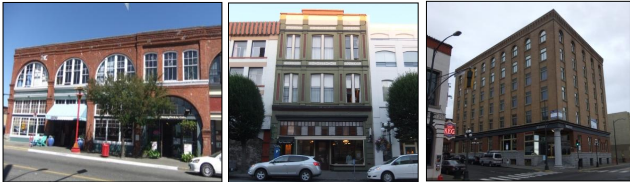
Figure 1 – Typical URM Buildings in Victoria
