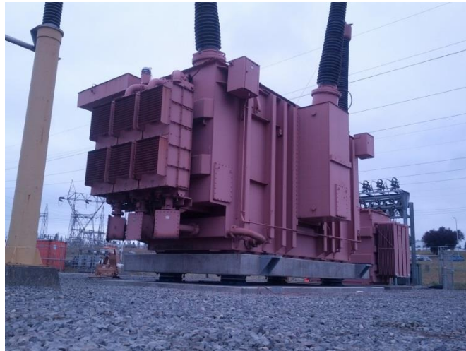
Figure 8, Completed Base Isolation Installation
