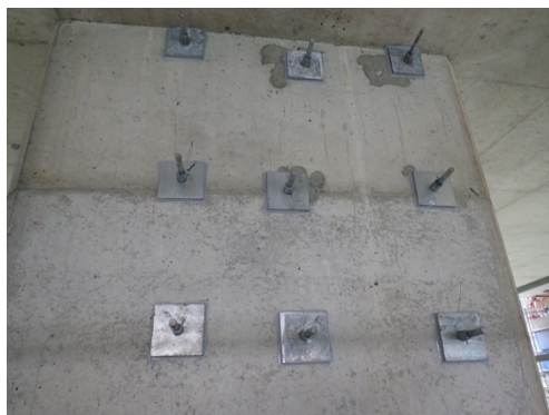
Fig. 4: West Pier Column Surface Anchors
