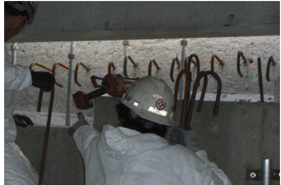
Fig. 5: Half-joint Diaphragm Rebar Being Placed
