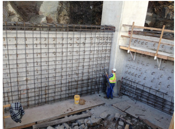
Fig. 3 – Typical Grade Beam Retrofit
