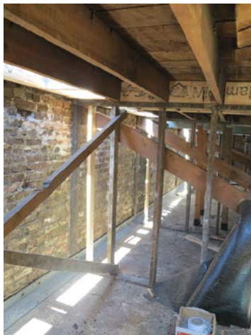
Fig. 5a (left) – Upgrading of Front Parapet on Marble Arch Hotel the angle to connect the brick to the diaphragm at the bottom of the parapet can be seen, plywood and connection at the top of parapet has not been performed at the time of the photograph.
