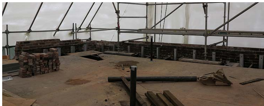
Fig. 5a (left) – Upgrading of Front Parapet on Marble Arch Hotel the angle to connect the brick to the diaphragm at the bottom of the parapet can be seen, plywood and connection at the top of parapet has not been performed at the time of the photograph.
