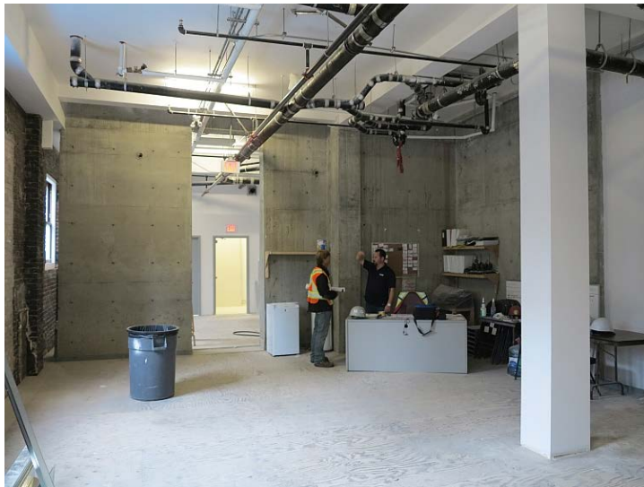
Fig. 2a (Left): Completed Concrete walls in the ground level of Marble Arch Hotel
