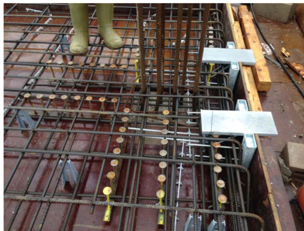
Figure 5: Reinforcing at a Typical Perimeter Column
