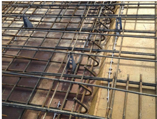
Figure 5: Internal Ties Hooking to PT at Transition in Slab Thickness
