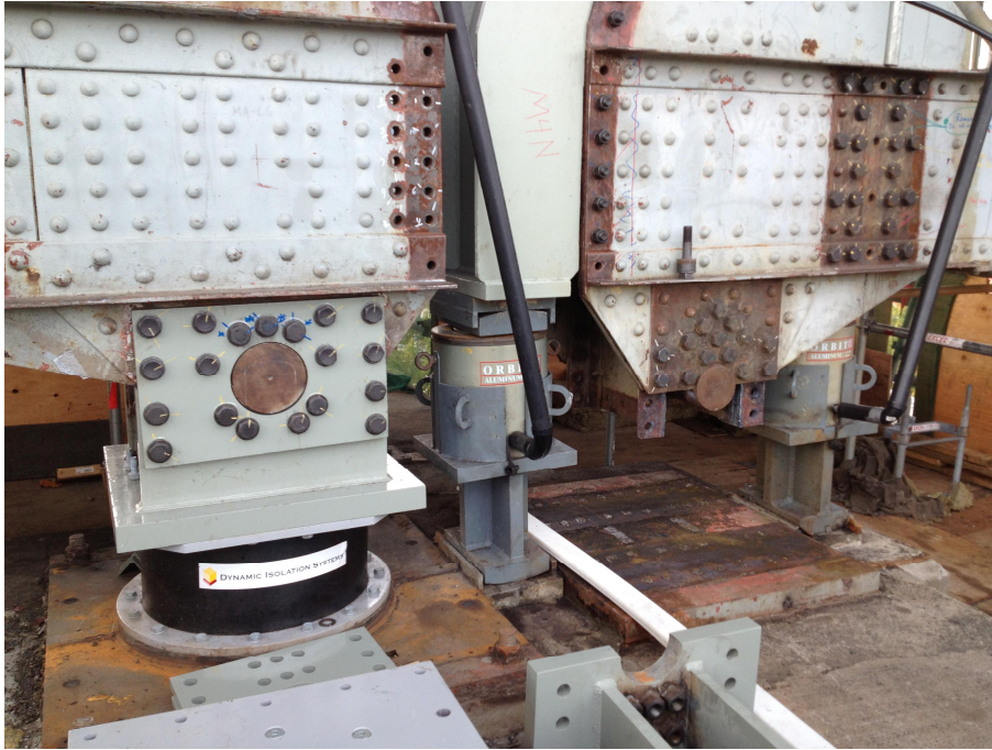
Fig. 8 – Completed Bearing Adjacent to Removed Bearing
