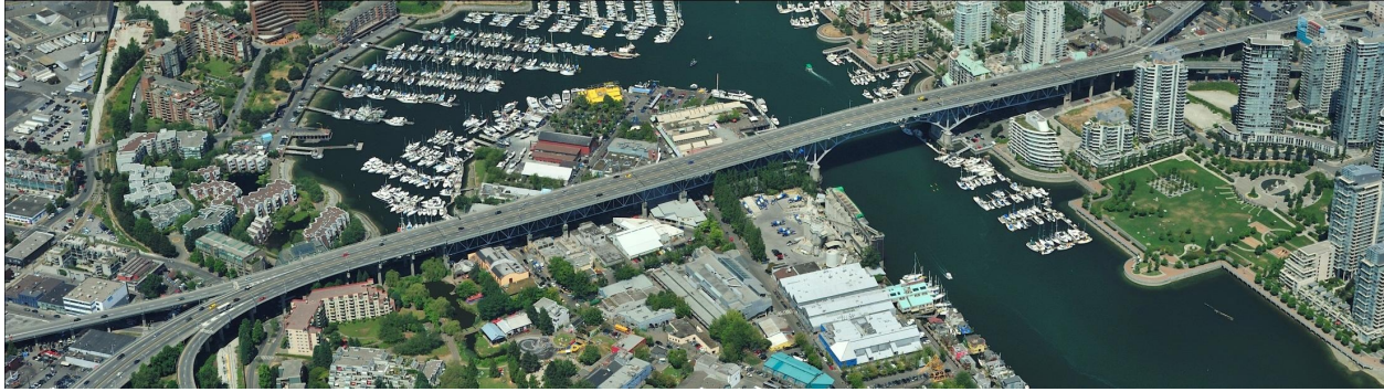
Fig. 1 – Aerial View of Granville Street Bridge (Looking West)
