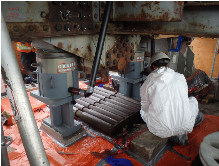
Fig. 7 – Preparing PCB Contaminated Rollers for Removal
