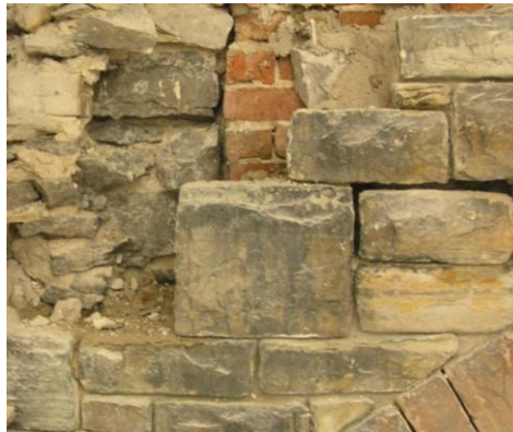
Coursed and uncoursed stone with different masonry in a wall.
