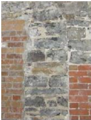
Mixed stone and brick masonry
