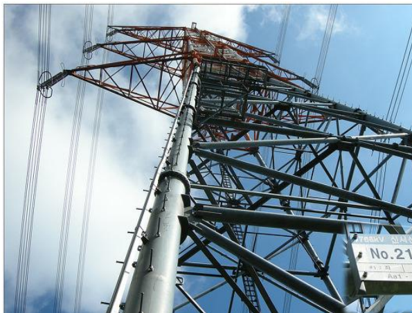
(a) Pipe-type transmission tower
