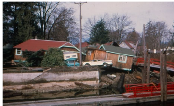
Fig. 2 – Damage at Port Alberni, BC in 1964 (Photo by D. Peregrine: CNN, 2007)
