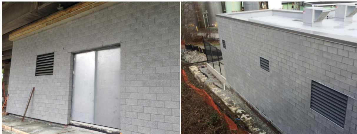
Fig. 7 – Substantial completion of Lougheed PPS (left) and North Portal PPS (right)
