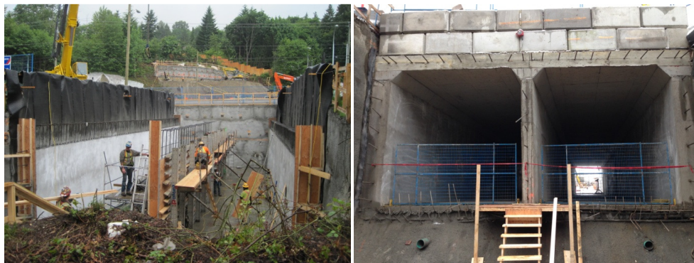
Fig. 7 – Construction of the Portal Tunnels
