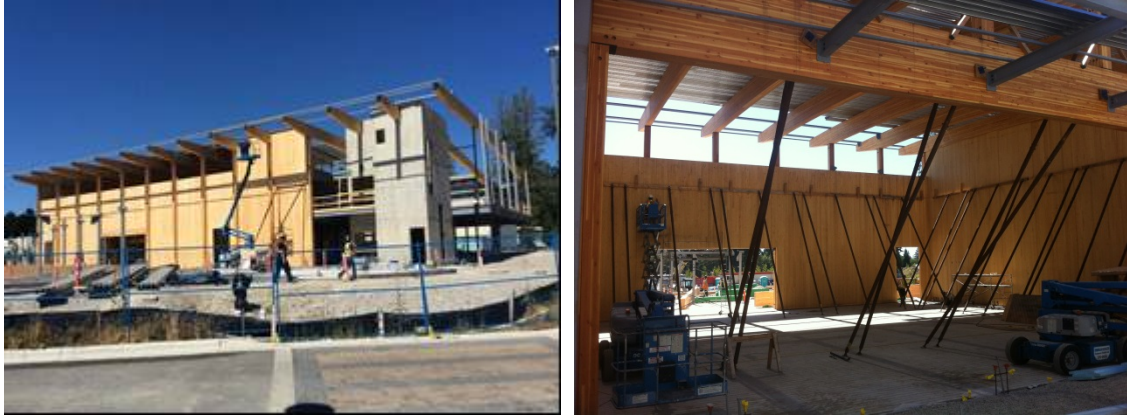
Fig 2. – Building under construction with CLT structural components in Vancouver, BC.
