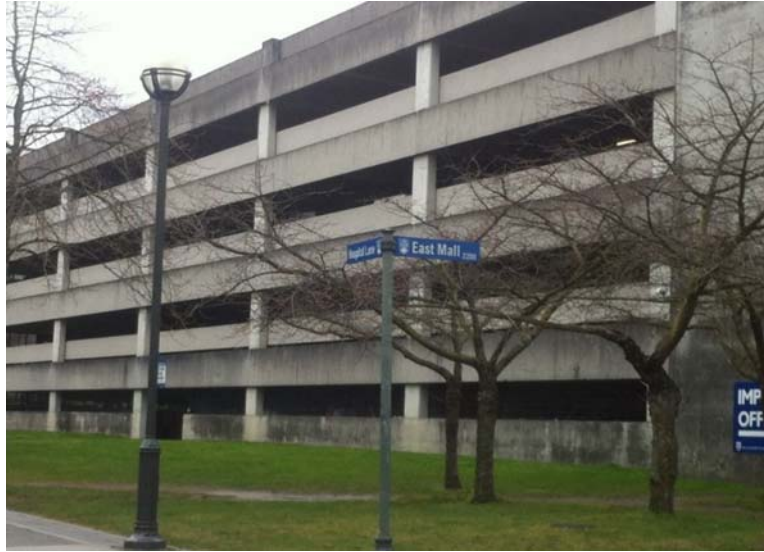
Figure 1: North Elevation of the Parkade.
