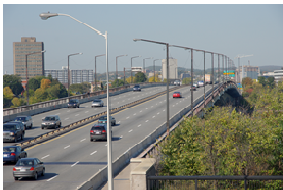
Fig. 1 – Aerial View of Macdonald Cartier Bridge
