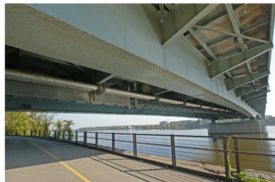
Fig. 2 – Steel Superstructure and Deck Soffit
