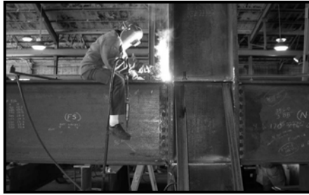
Simulated Pre-Northridge Field Welding
