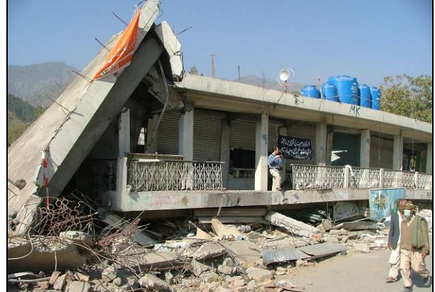
Figure 3. Structural failures due to soft story along main street in Balakot.
