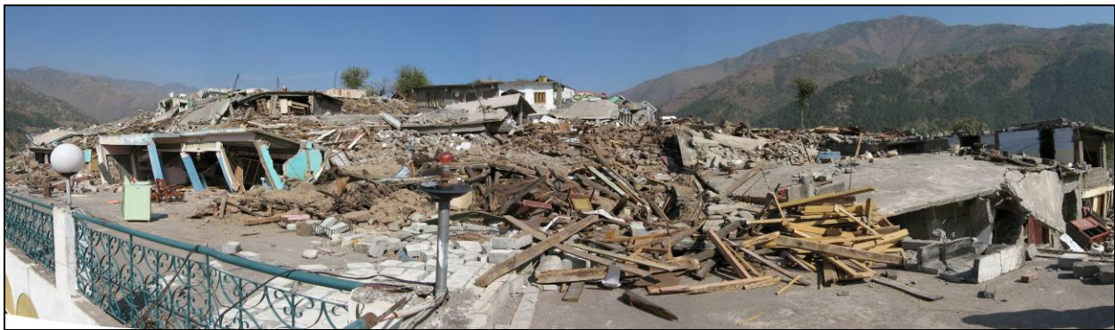
(a) Pictorial view of ridge effect on collapse on a hill in Balakot.
