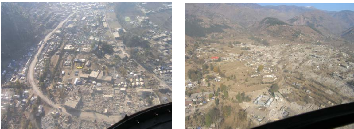
Figure 3. Aerial view of damage around Muzaffarabad.
