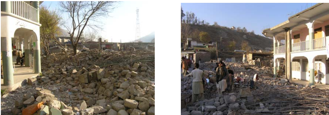
Figure 6. Collapsed un-reinforced masonry buildings in Balakot.
