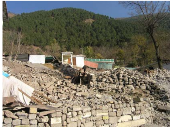
Figure 5. Collapsed Stone houses in Balakot.
