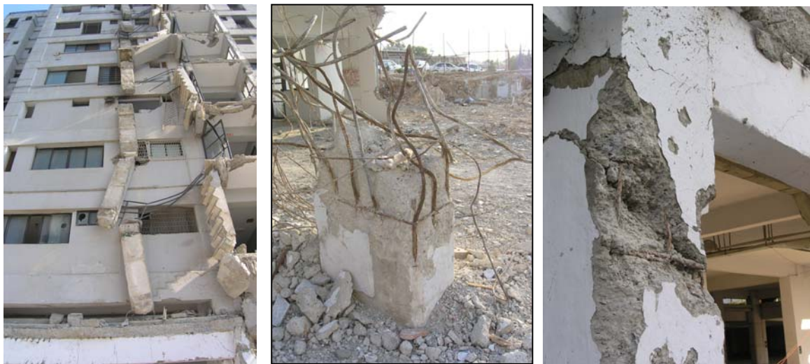
Figure 13. Structural and reinforcement details in Margala structures.
