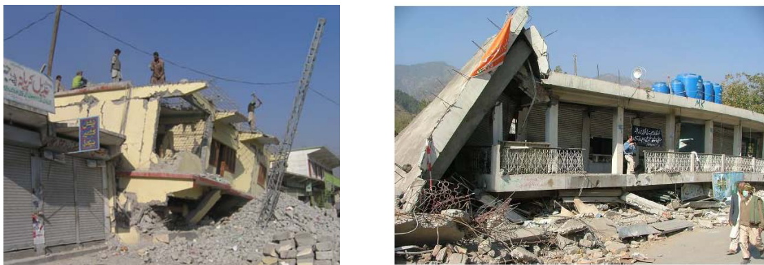
Figure 9. Soft storeys in buildings in Muzaffarabad and Balakot (Durrani et al 2005).
