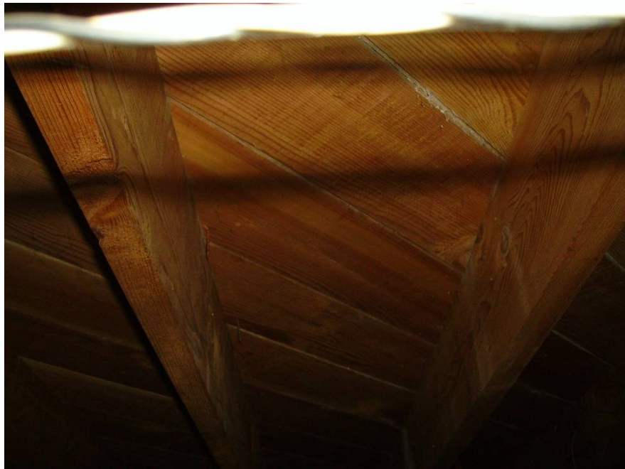
Typical floor structure, diagonal shiplap over joists
