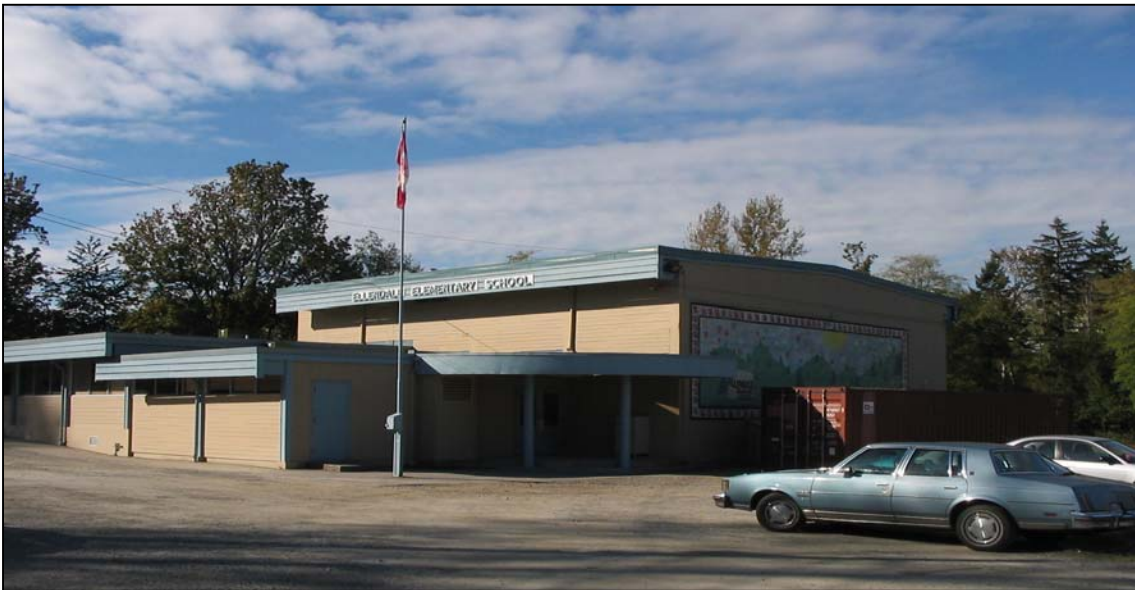
Front of Ellendale Elementary School Looking at the Gymnasium.
