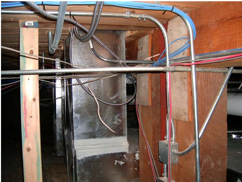
Picture 5 Crawlspace under Classroom Block
