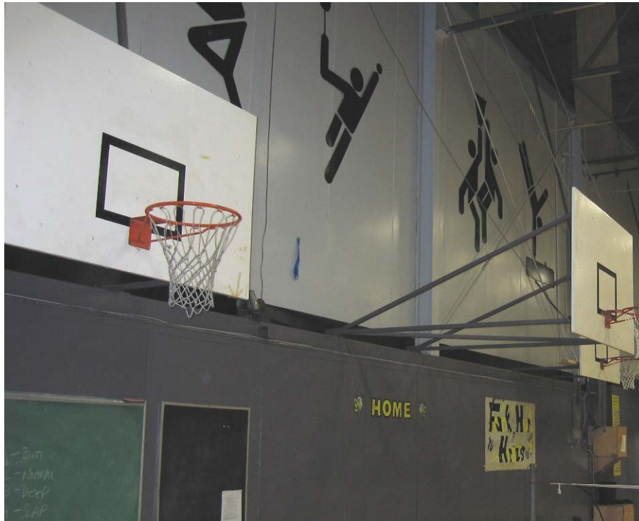
Figure 3 Interior View of Braced Bay
