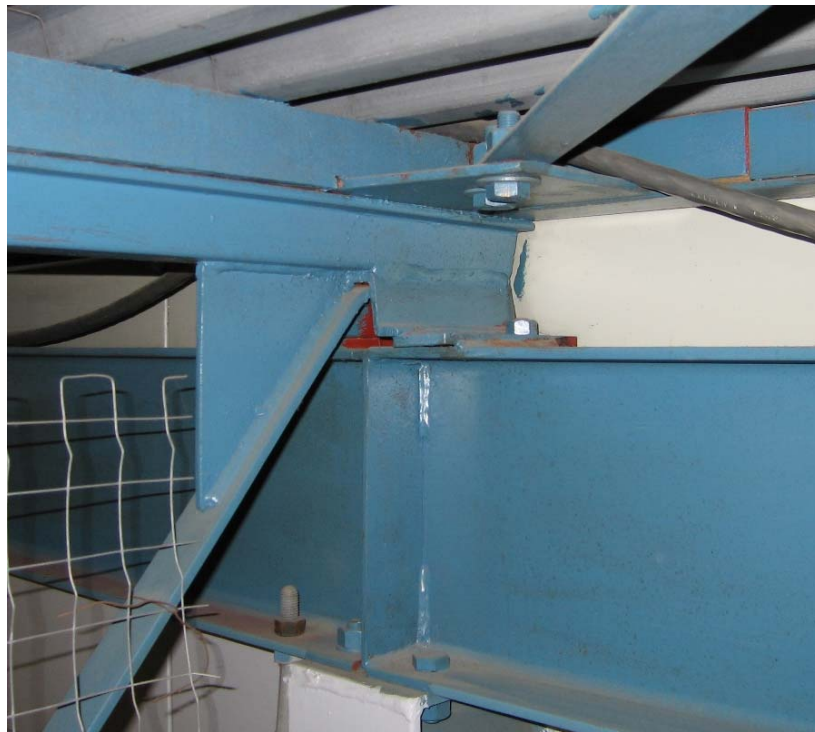
Figure 2 Roof Connection Details
