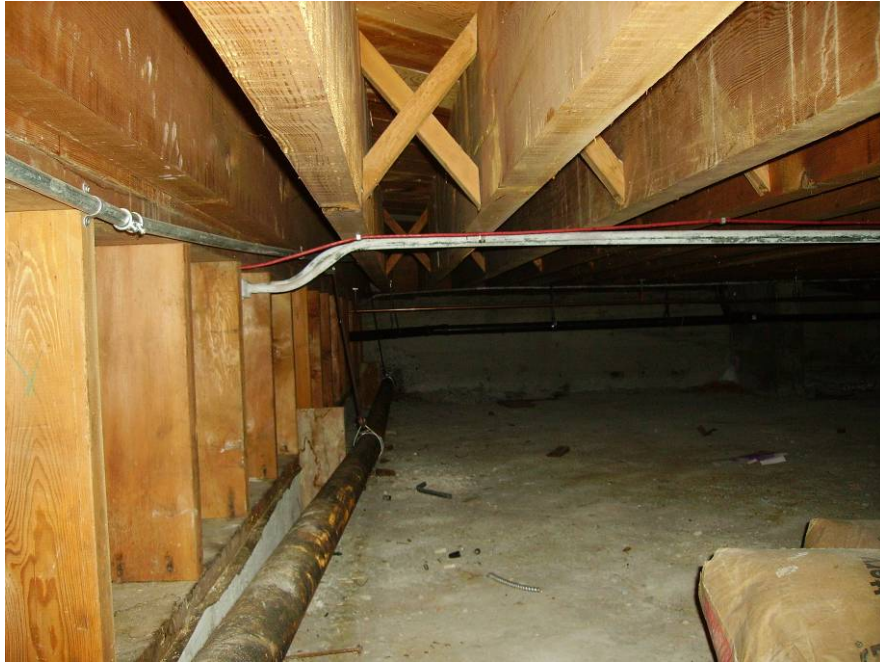
Crawl space area, typical pony wall under load bearing partition wall
