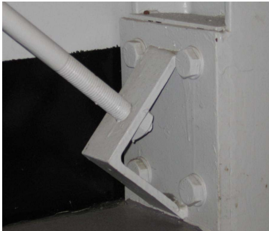
Figure 4 Existing Braced Bay Connection
