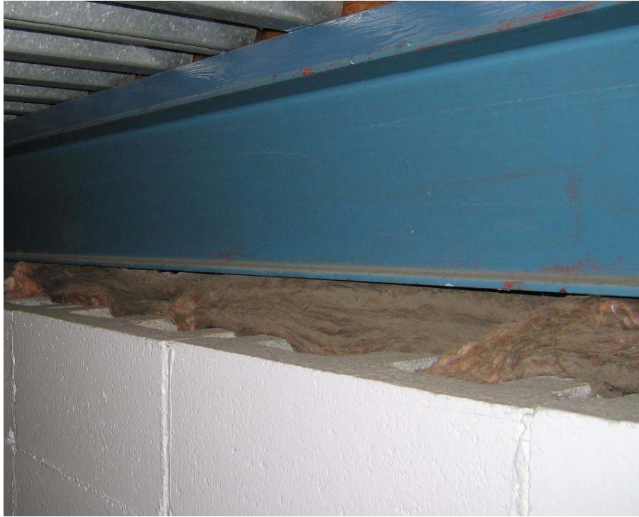
Figure 5 Top of Existing Masonry Wall
