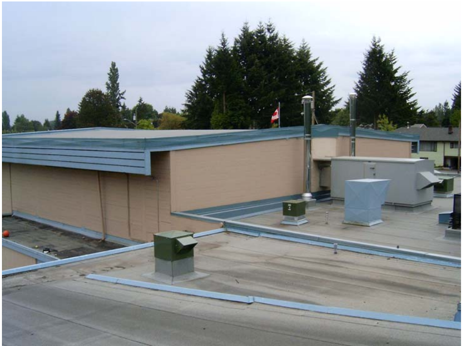
Picture 2 Exterior View of Roof
