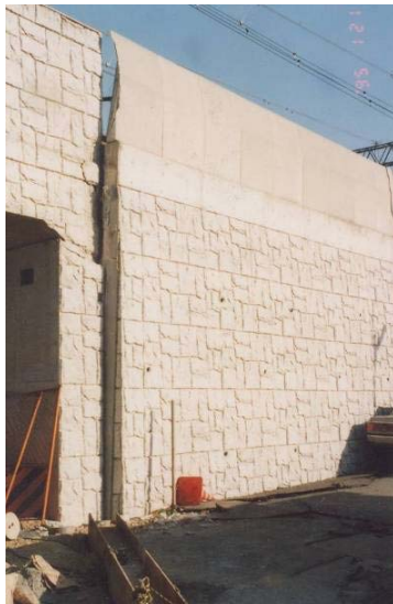
a) Tanata wall showing 10 cm movement at base
