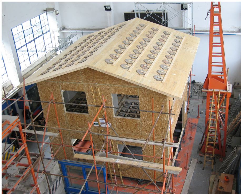
Figure 2. View of test specimen 1.
